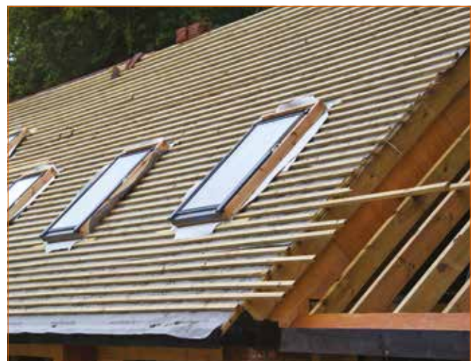
Being a structural product, battens should be properly graded
